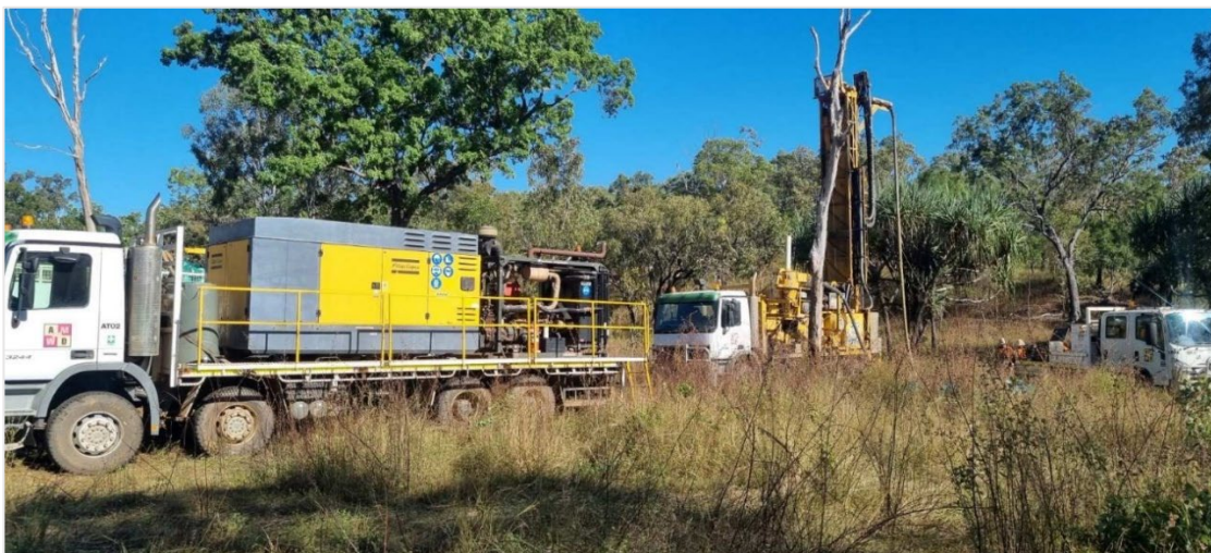
Figure 1: AMWD drill rig setting up at Leliyn Graphite Project
