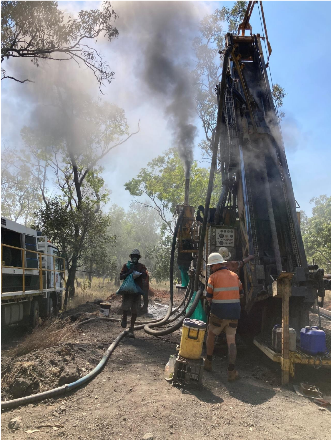
Figure 1: AMWD drill rig drilling LERC_08
